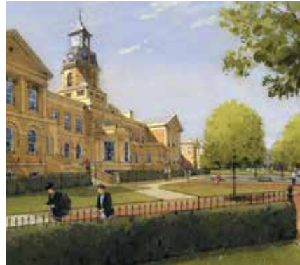
Refurbished Cambridge Military Hospital
